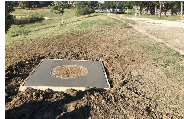
Eastern Hills Manhole
