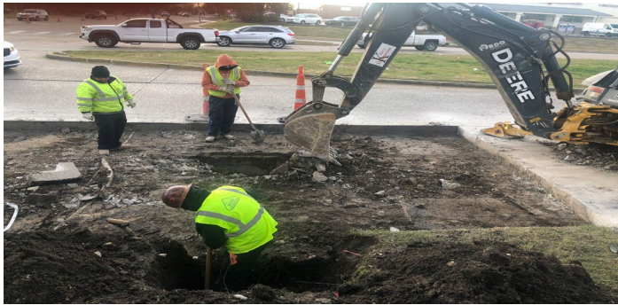
Clifford Storm Drain Repair
