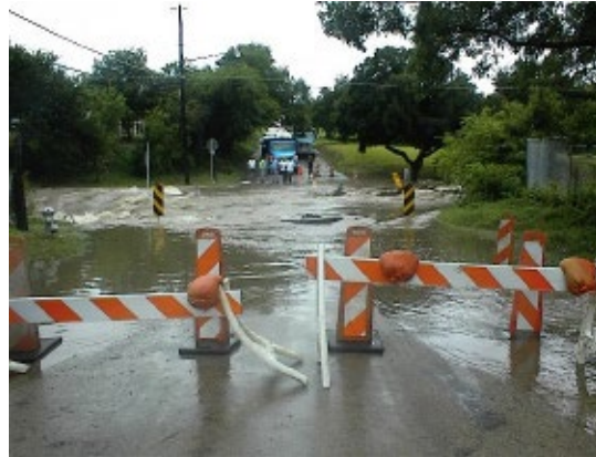
June 2004: E. Butler St. & McClure St. Flooding
